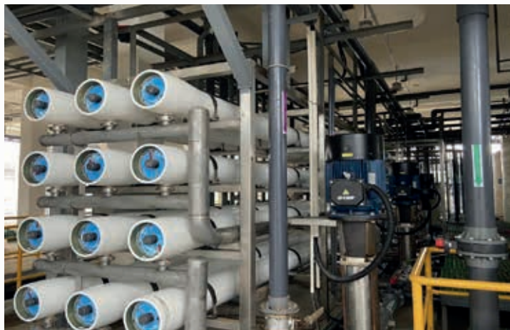
Figure 1 Water Recycling System at the Eco-plating Specialised Zone 圖1 環保電鍍專業區內的水循環系統
